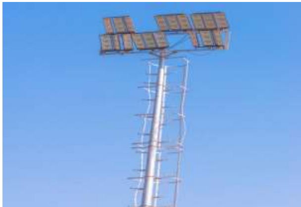
High Mast Pole
